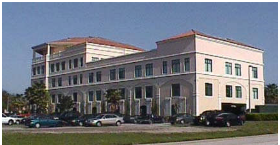
VIEW NORTH FROM PARK CENTER DRIVE
