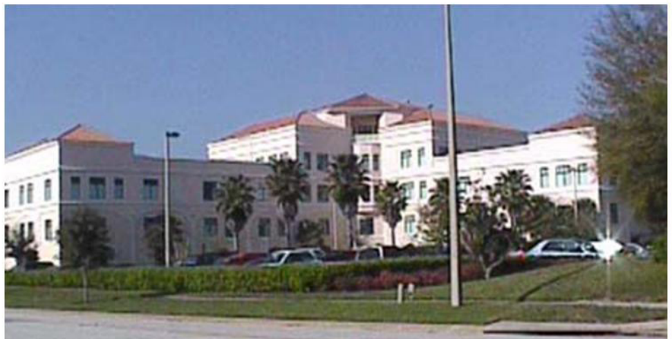
VIEW SOUTH FROM PARK CENTER DRIVE
