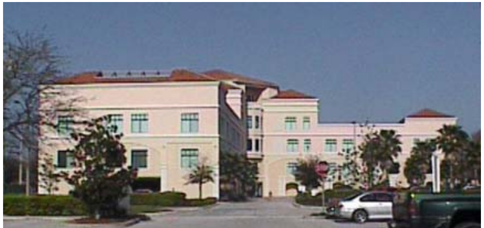
VIEW WEST FROM PARK CENTER DRIVE
