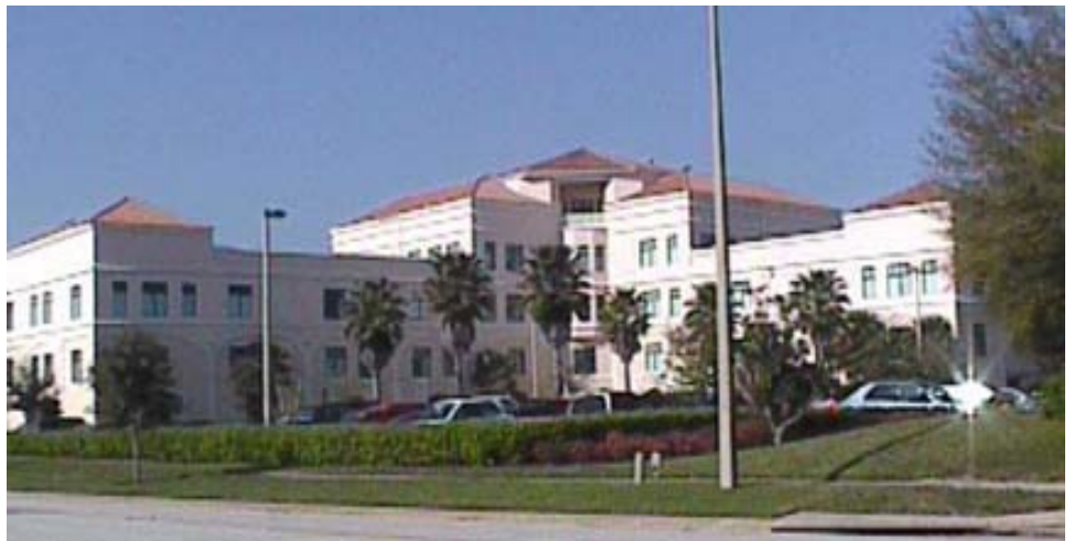
VIEW SOUTH FROM PARK CENTER DRIVE
